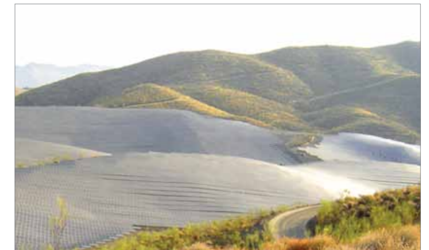
Xantrex GT500 E installation at Almería, Spain.
